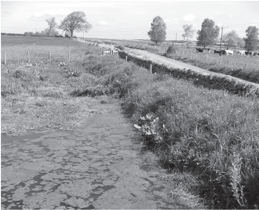
Fig. 19.9 Field corner storage pond at Nafferton Farm, managed by Newcastle University. Runoff from the field above is collected in the pond, which discharges into surface water drains to the right of the photograph.
